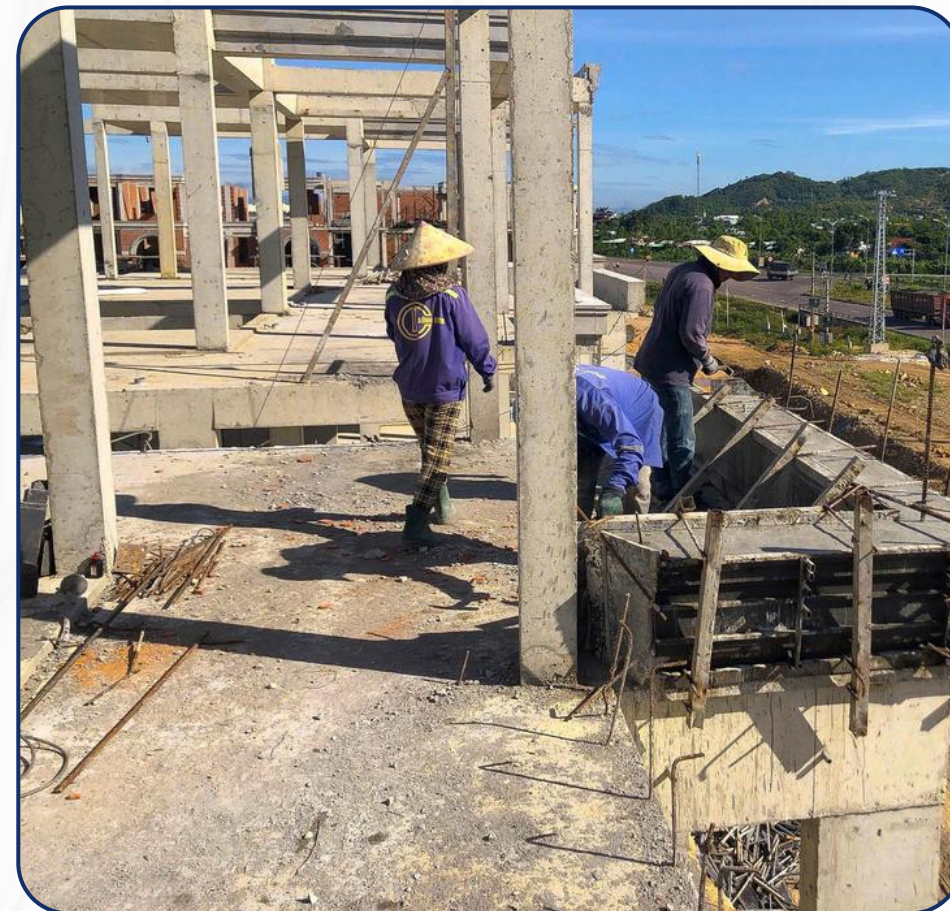
Finalizing the in-house utility parks
