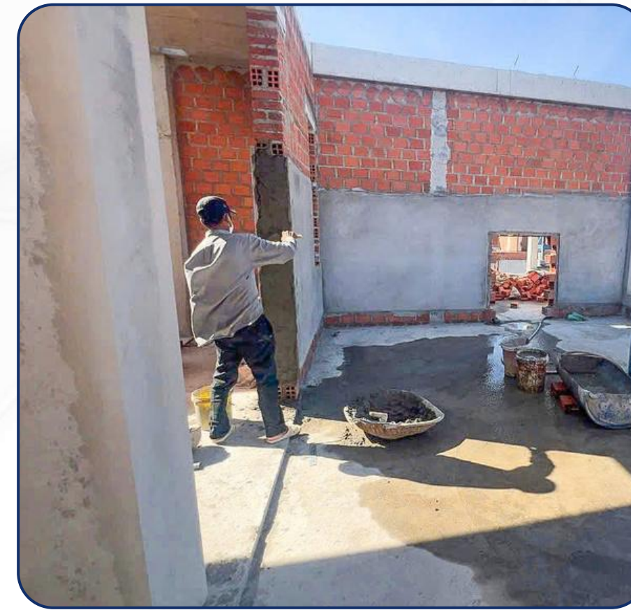
Actively pouring concrete slabs for shophouse rows
