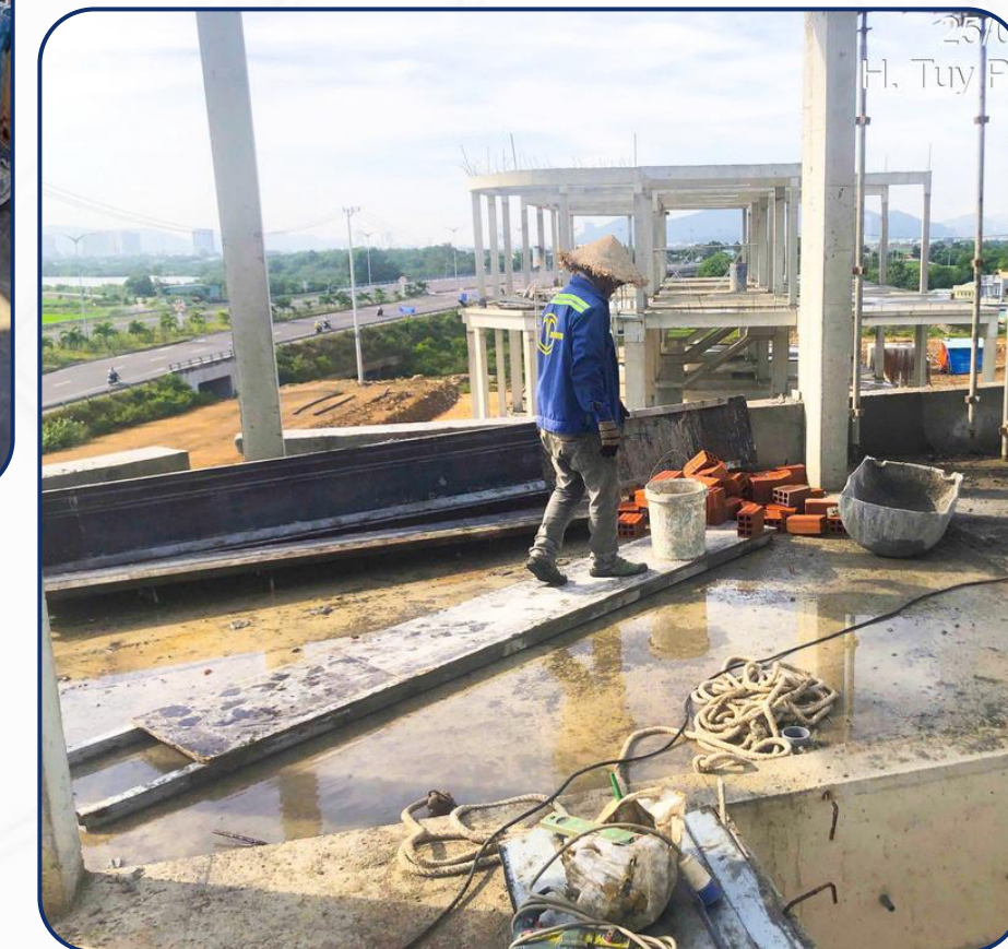
Completing shophouses facing National Highway 19
